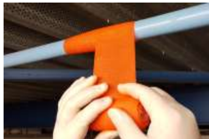
2. Apply Wrap Repair
